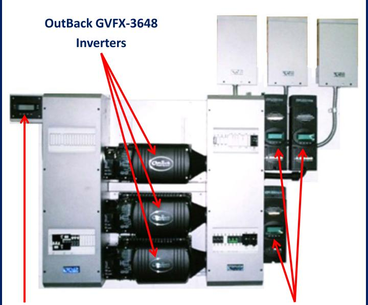
Mate2 System Display and Controller OutBack FM-80 Charge Controllers
